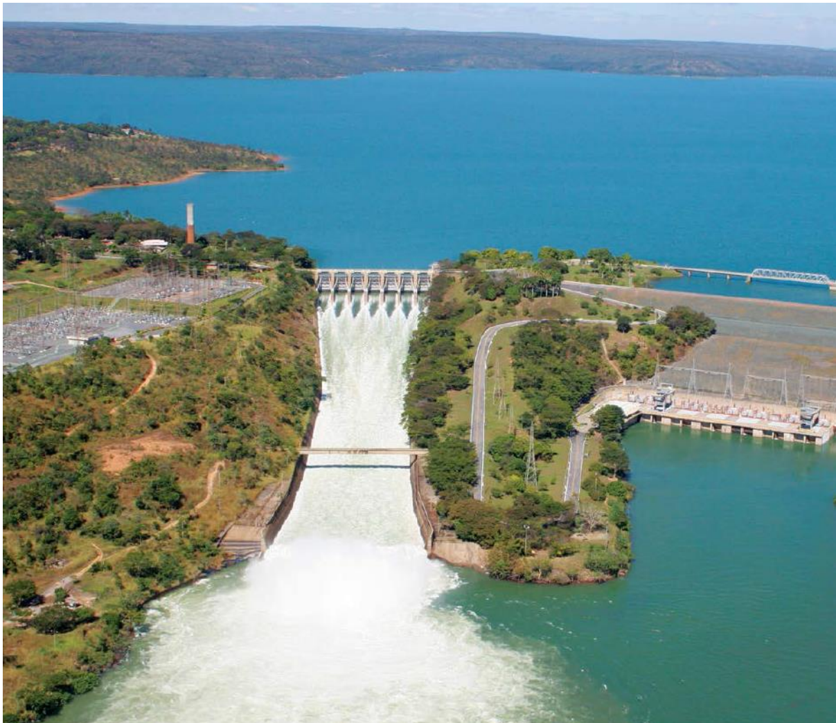
Três Marias Dam spillway (Picture published with the friendly permission of CEMIG)
